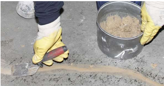
Figure 5. Levelling the crack surface by using proper MasterBrace mortar.
