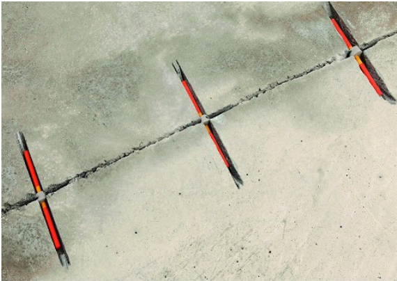
Figure 3. Placing the screed ties into the canals opened on the cracks.
