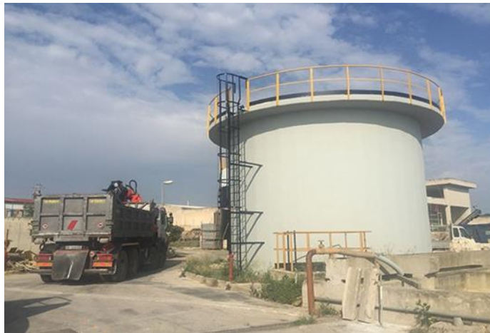
Application of MasterSeal M 689 polyurea waterproofing and protection membrane.
