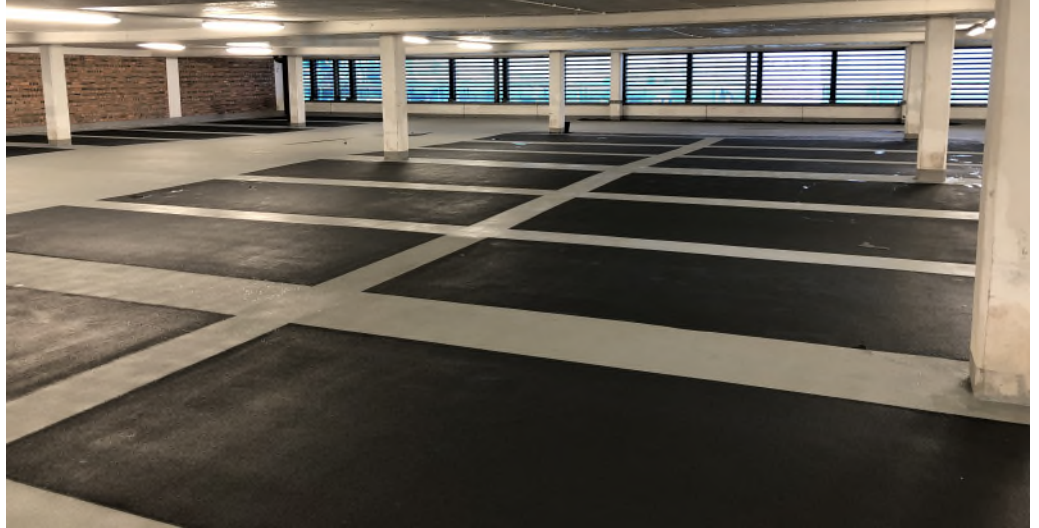
Our reference in Glasgow (United Kingdom), Waterloo Street MSCP
