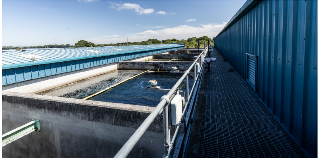
Our reference in Northern Ireland (United Kingdom): Water Treatment Works
