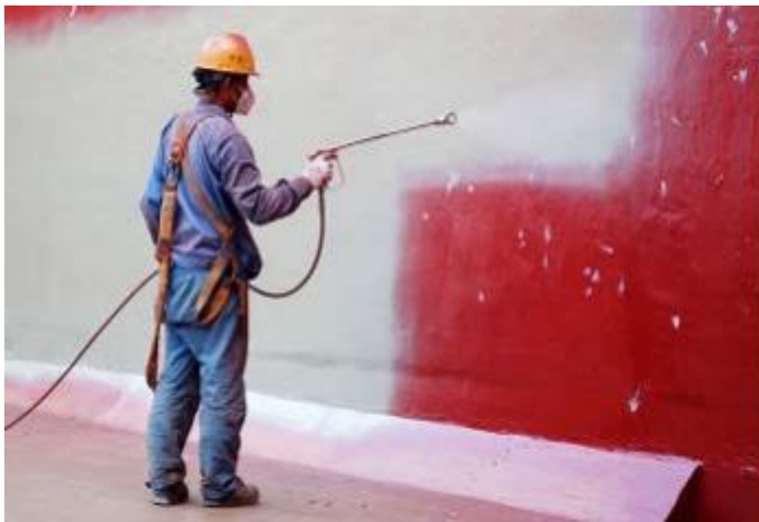
MasterSeal 7000 CR is available in 2 colors – red and grey, for easy identification from first and second coat event in environment with poor visibility.
