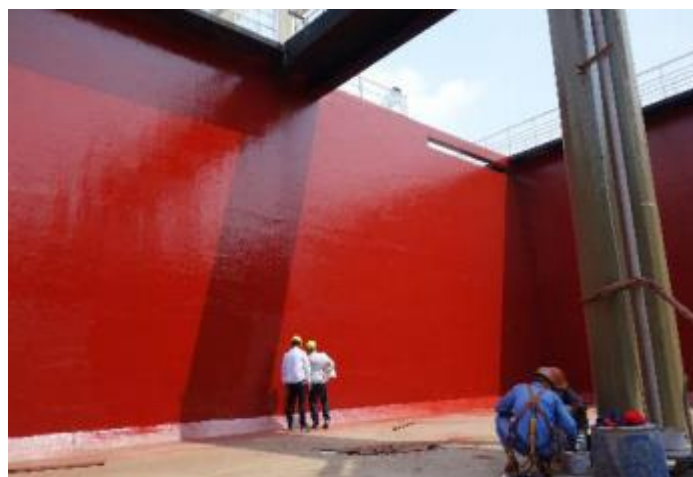
MasterSeal 7000 CR can be applied easily, either by spray or roller.
