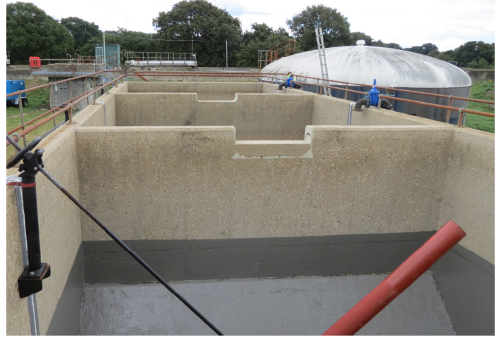
Our reference in Southampton (United Kingdom): Sewage Water Treatment Works
