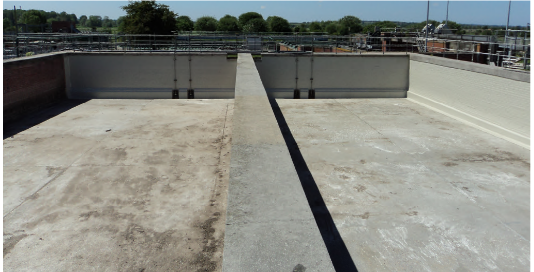
Our reference in Glastonbury (United Kingdom): Sewage Treatment Works
