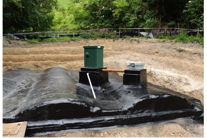
Our reference in Sussex (United Kingdom): Coombe Down Reservoir Roof
