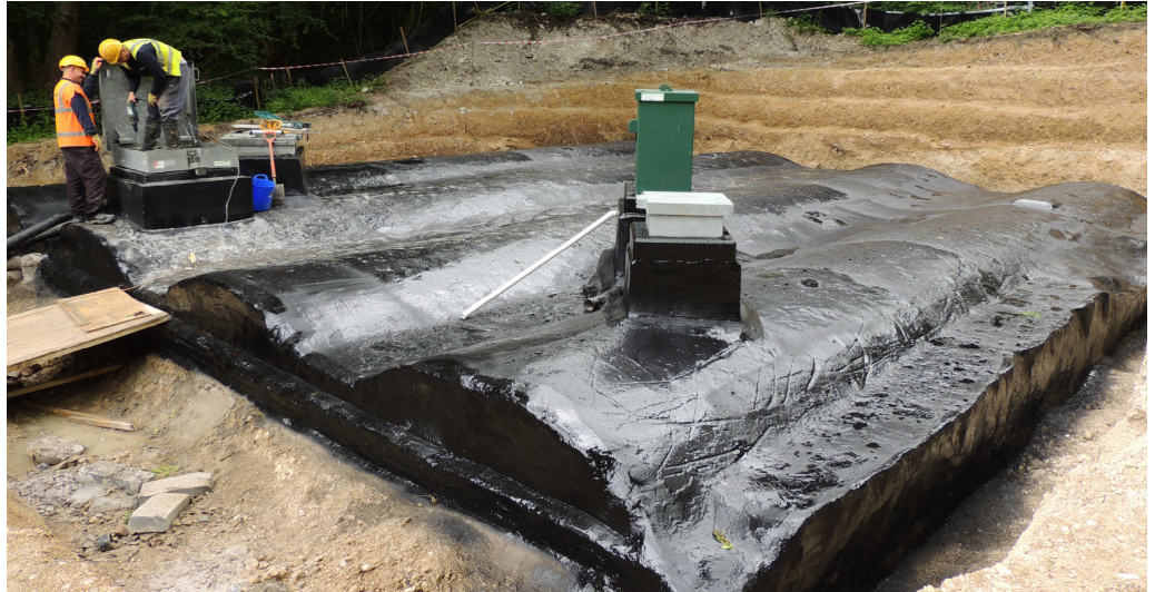
Our reference in Sussex (United Kingdom): Coombe Down Reservoir Roof
