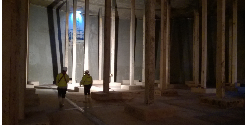
Our reference in East Sussex (United Kingdom): Service Reservoir
