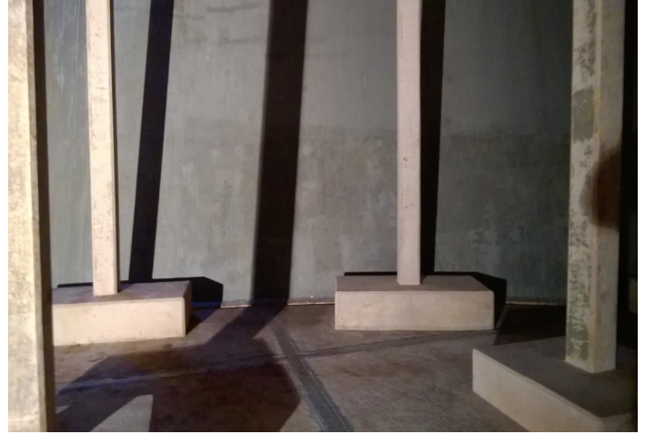
Our reference in East Sussex (United Kingdom): Service Reservoir
