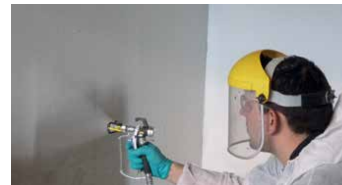
Spray-application of MasterProtect 330 EL as crack-bridging anti-carbonation protection of a car park wall.
