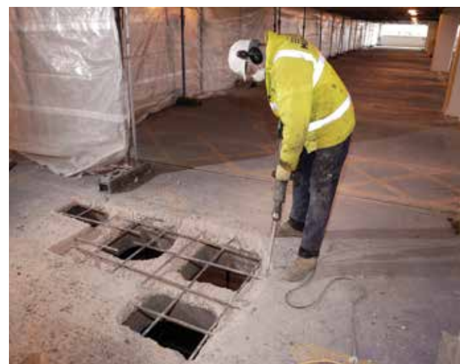
Cut out preparation, full depth repair.
