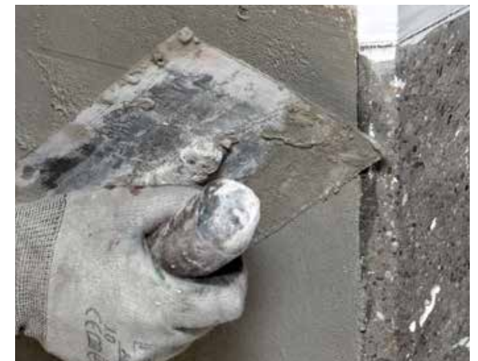
Levelling of surface with MasterEmaco N 5100 FC
