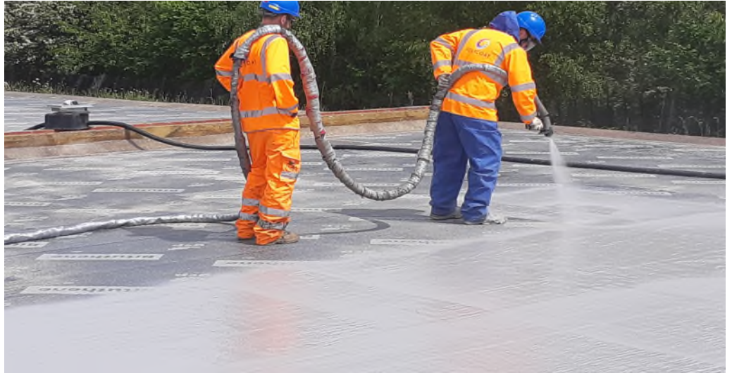
Our reference in West Sussex (United Kingdom): Reservoir Roof
