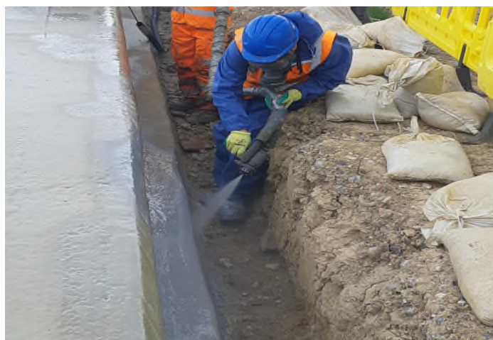
Our reference in West Sussex (United Kingdom): Reservoir Roof
