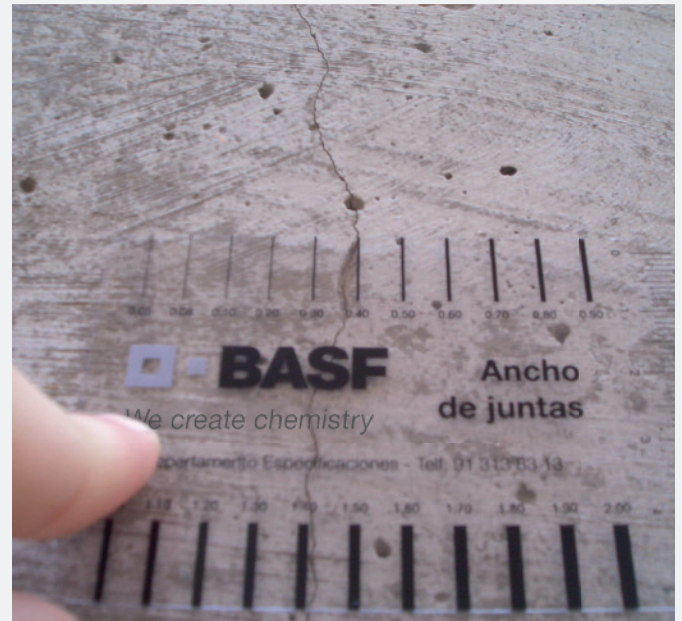
Hairline cracks
