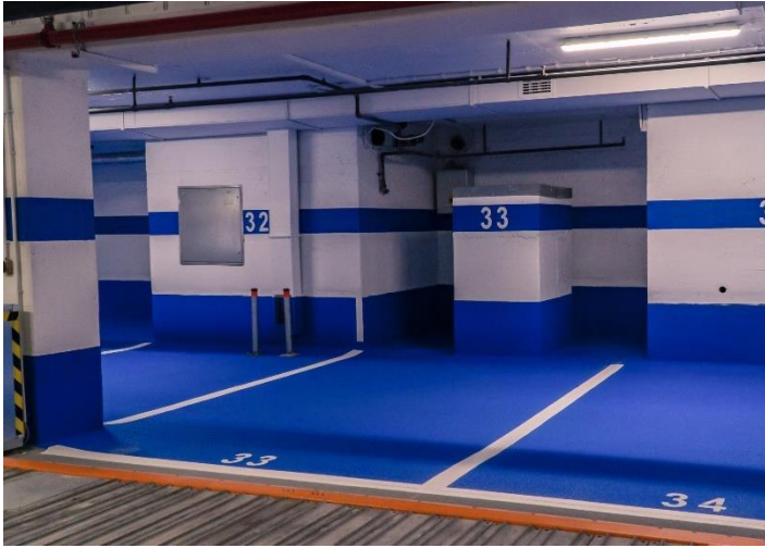
MasterSeal Traffic 2239 was used on the underground decks and MasterSeal Traffic 2219 on the ramps and the inner courtyard
