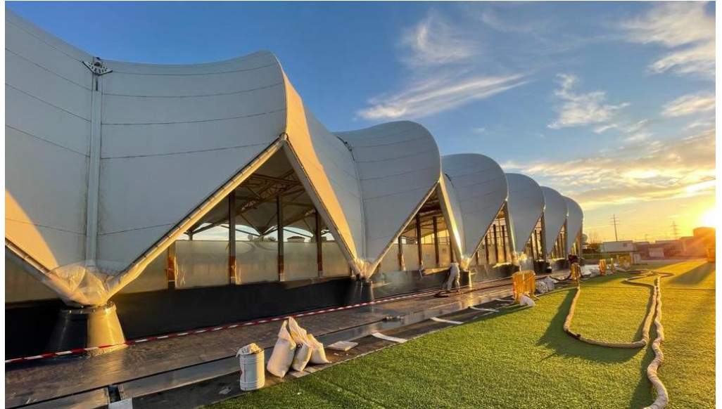
MasterSeal Roof 2111 waterproofing on sport area in UNEATLANTICO in Santander, Spain.
