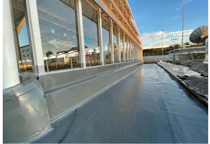
MasterSeal Roof 2111 waterproofing on sport area in UNEATLANTICO in Santander, Spain.
