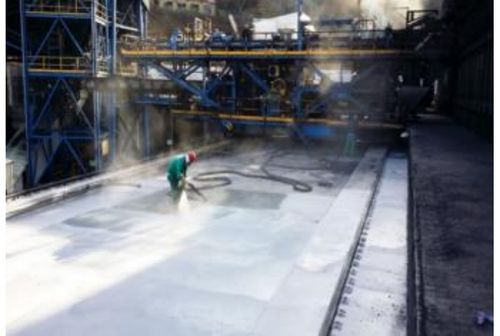
Spraying of MasterSeal M 689 polyurea membrane
