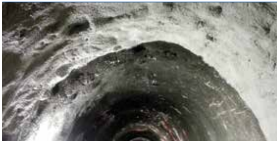
Cordee Montblanc tunnel (Italy)
