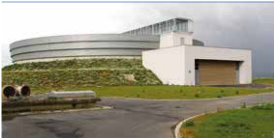
Tank for potable water
