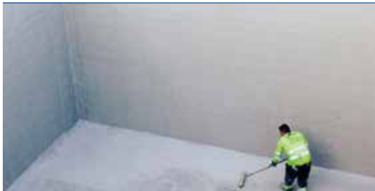
Process water reservoir, Montejo (Salamanca - Spain)
