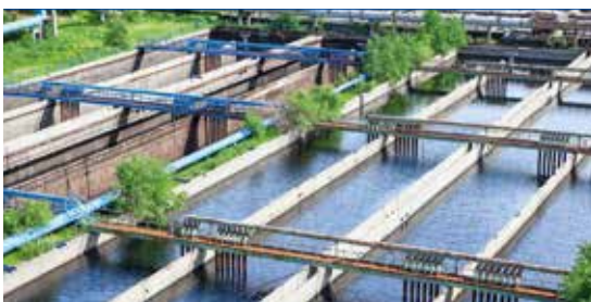
Tank for industrial process water
