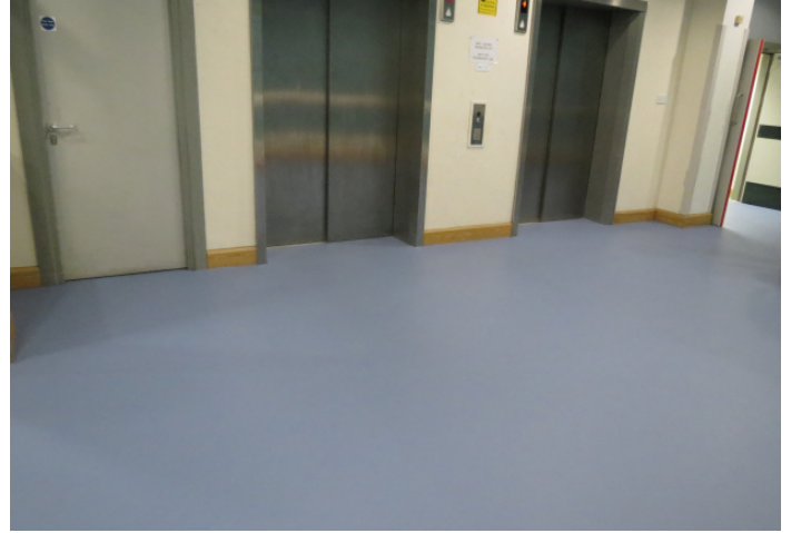
Our reference in Gloucester, United Kingdom: Gloucestershire Royal Hospital
