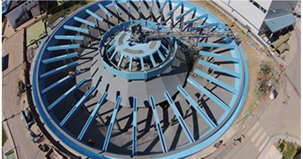
Aerial view of the primary sedimentation tank at the water treatment works ETAP El Atabal, (Málaga – Spain)
