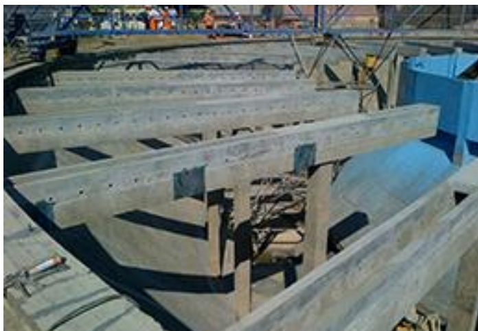
Full refurbishment including concrete repair, reinforcement, and protective waterproofing in accordance with EN 1504
