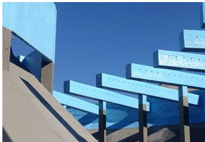
Full refurbishment including concrete repair, reinforcement, and protective waterproofing in accordance with EN 1504
