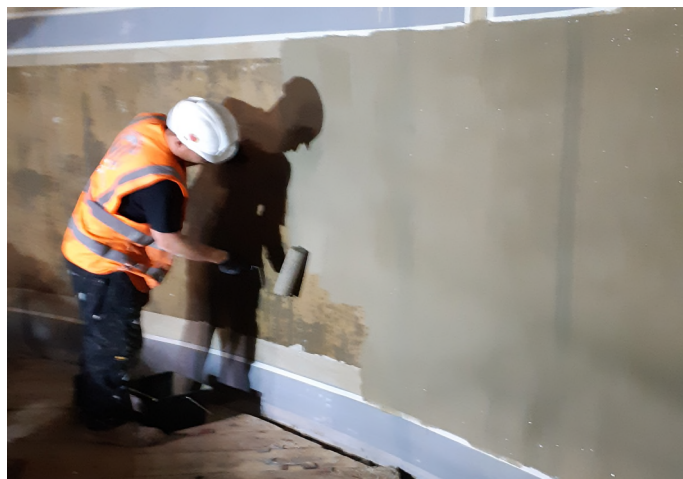
Our reference in Kidderminster (United Kingdom): Digester refurbishment
