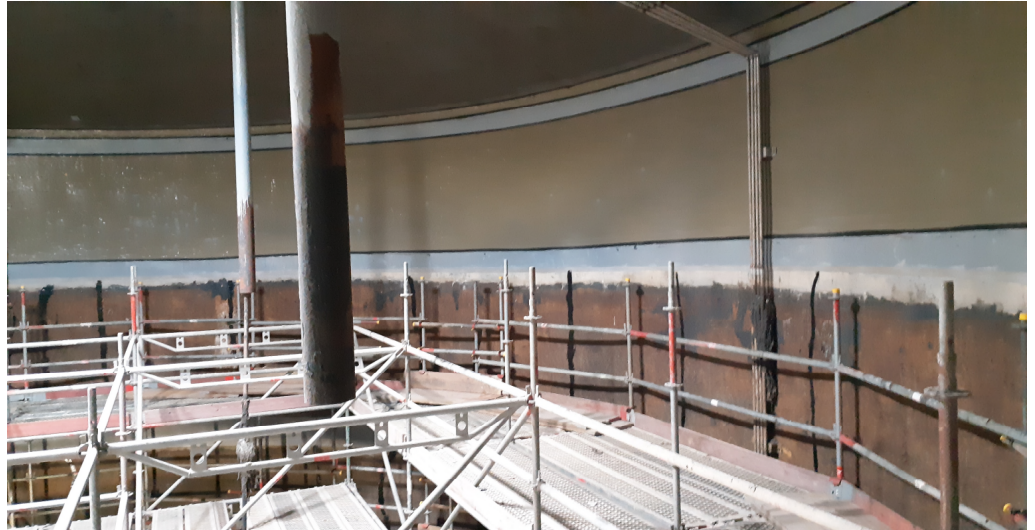
Our reference in Kidderminster (United Kingdom): Digester refurbishment
