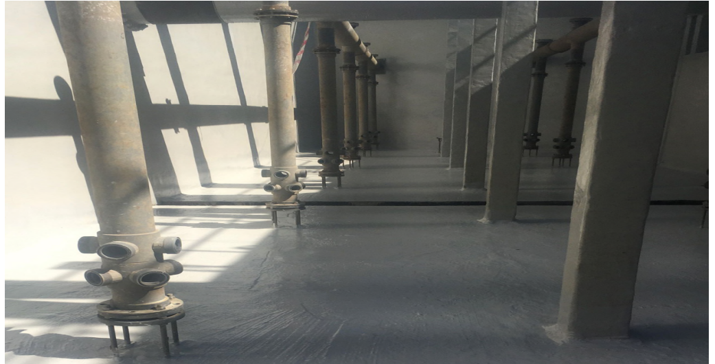
Our reference in Northumbria (United Kingdom): Clarifier refurbishment
