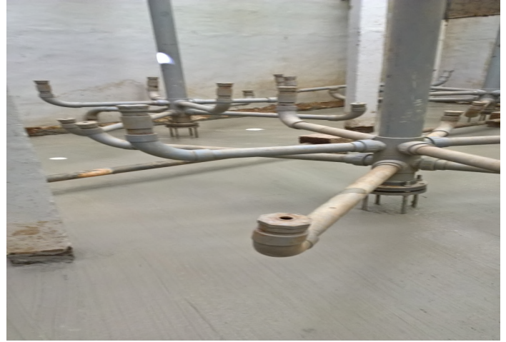
Our reference in Northumbria (United Kingdom): Clarifier refurbishment
