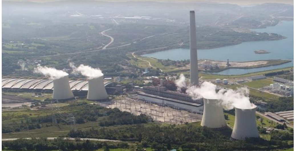
General view of the thermal power plant
