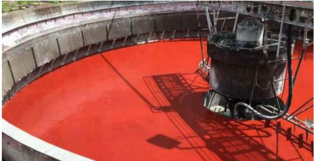
Tank refurbishment and waterproofing
