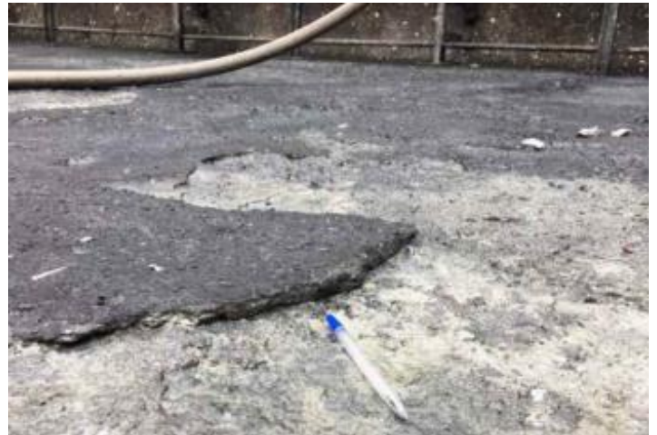
Tank refurbishment and waterproofing
