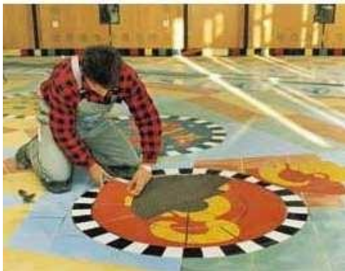
Secure laying of tiles with Mastertile FLX 23
