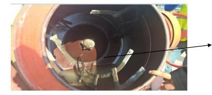
Flowable grout MasterFlow 524 will obtain that will pour through the upstand shutter with 45 degree that form the desired slope for grouting under this big machine
