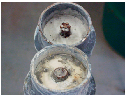
With corrosion inhibitor
