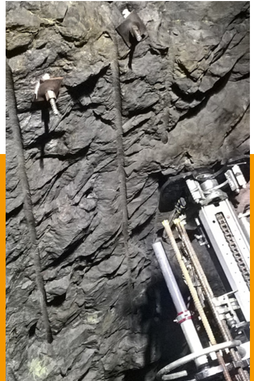
Self-drilling anchor with MasterRoc RBA 380
