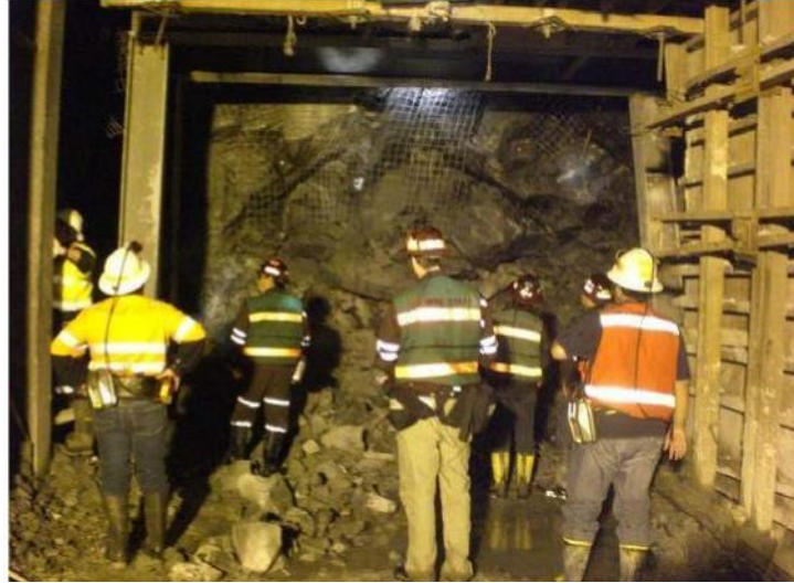
Our reference in Ground collapse at Freeport underground mine production area. Location at panel 5, Deep Ore Zone underground mine.
