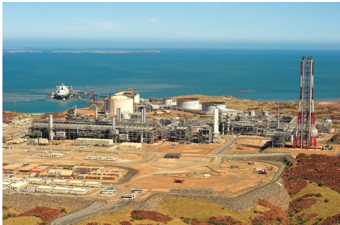
Pluto LNG onshore gas plant. Source: Woodside image gallery
