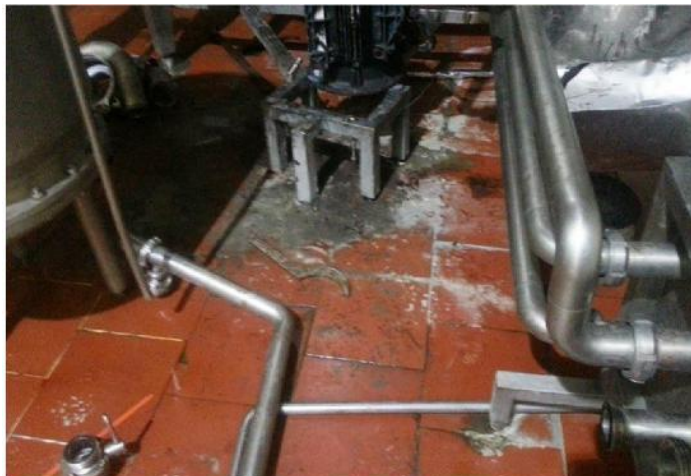
Flooring condition before application of Ucrete
