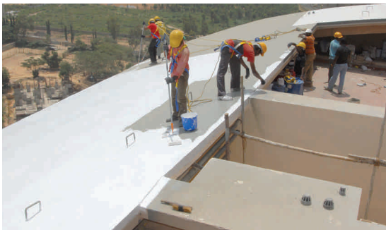
MasterSeal Roof 3500 Brigade condominium, India
