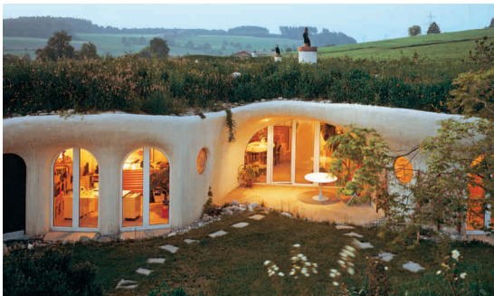
MasterSeal Roof 3000 Roof garden on private home, Switzerland
