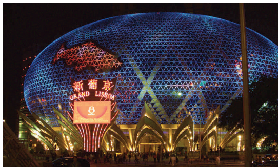
MasterSeal Roof 3500 Grand Lisboa, Macau
