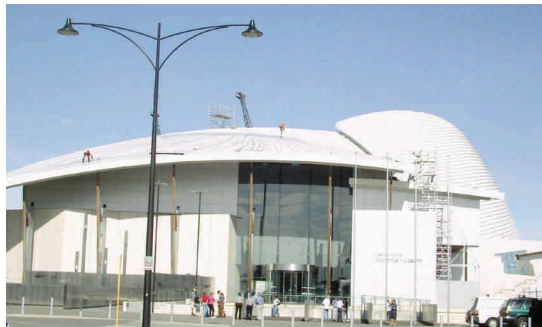
MasterSeal Roof 3500 Maritime Museum, Western Australia
