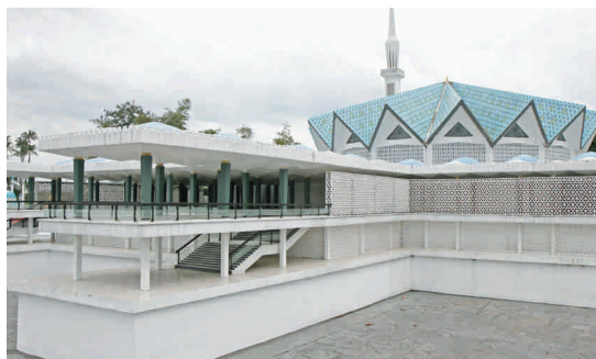
MasterSeal Roof 3500 National Mosque Kuala Lumpur, Malaysia
