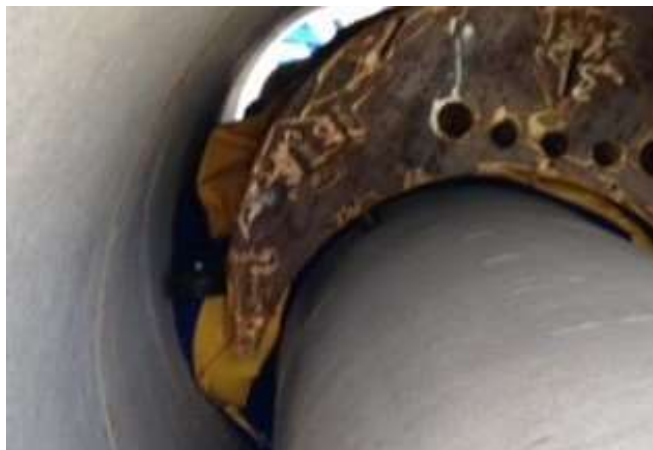
Mock-up inflatable bags before filling with precision grout
