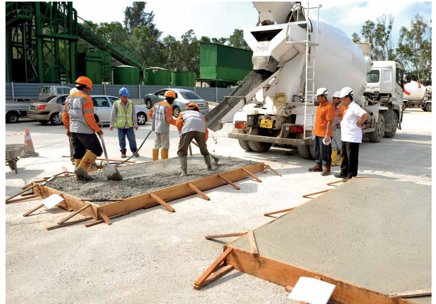
One of the greatest benefits for constructors and builders is higher productivity in the concrete placement process. The ease of application requires less manpower and reduced claims for defects, voids and honeycombs.
