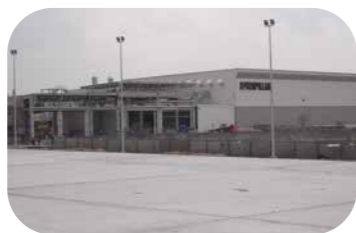
Caterpillar Production Distribution Center, Thailand
