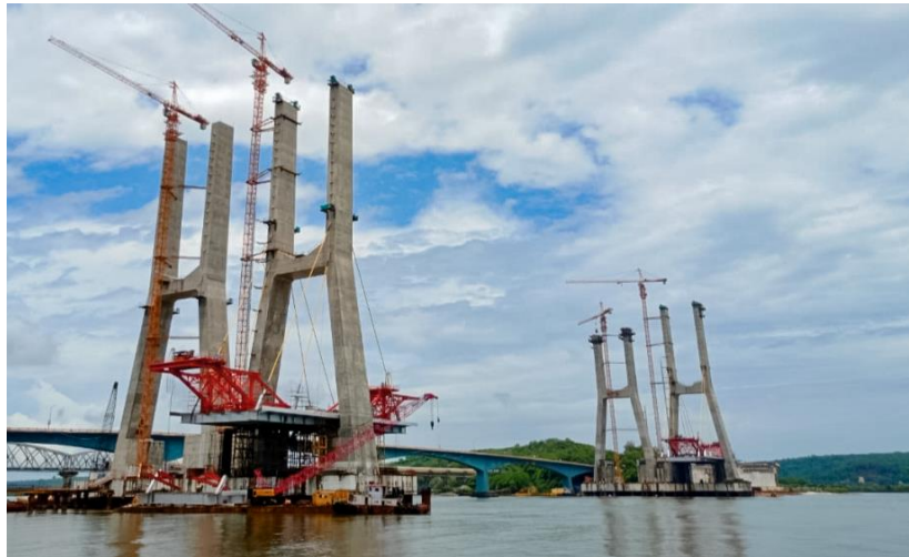
Our reference in Goa (India): Zuari Cable Stayed Bridge
