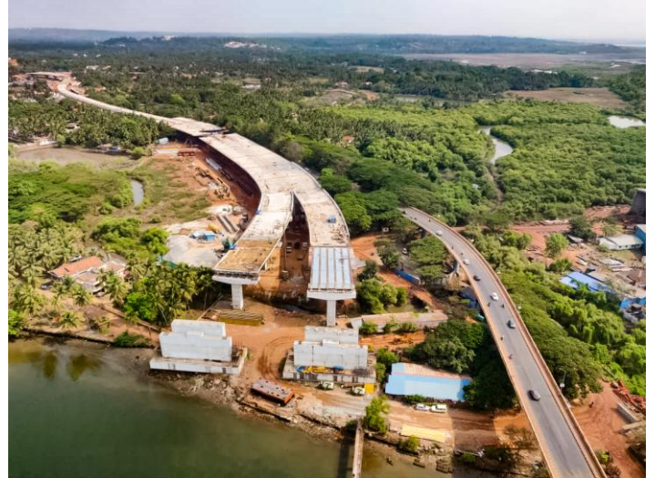
Our reference in Goa (India): Zuari Cable Stayed Bridge
