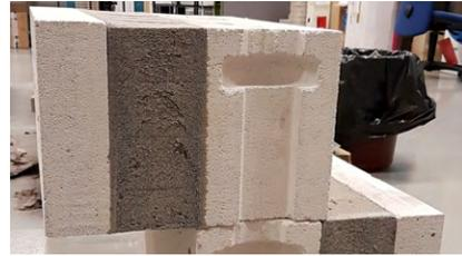
Example of insulated double-layer masonry. MasterProtect NFF 2000 IN insulates the wall and holds the facing formwork without reinforcement.
