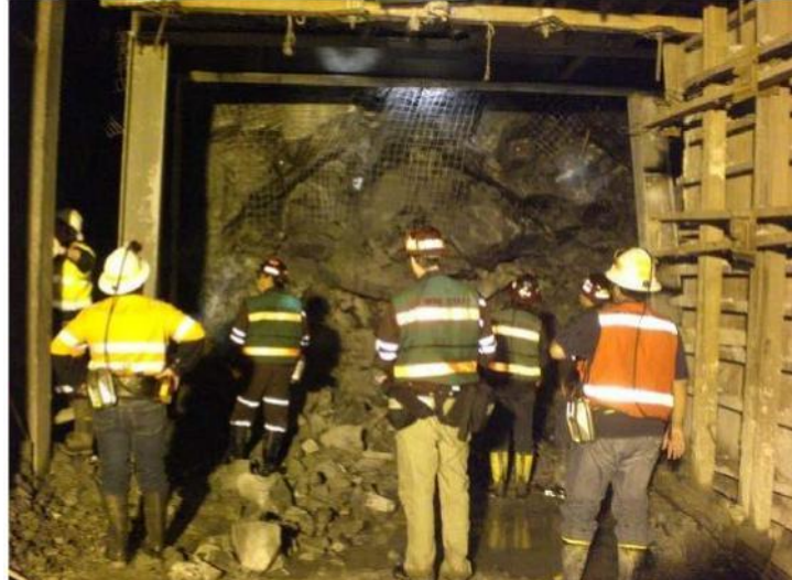
Our reference in Ground collapse at Freeport underground mine production area. Location at panel 5, Deep Ore Zone underground mine.
