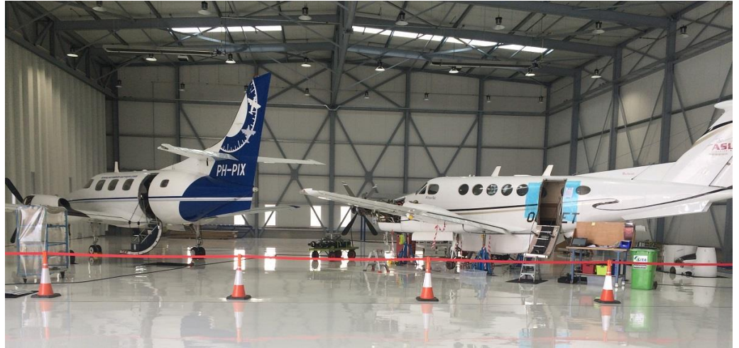
Onze referentie in Rotterdam (Nederland): The Hague Airport hangar
