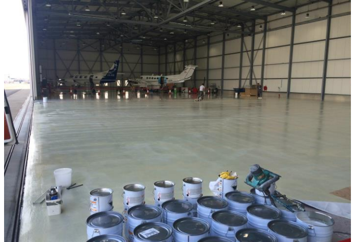
Onze referentie in Rotterdam (Nederland): The Hague Airport hangar
