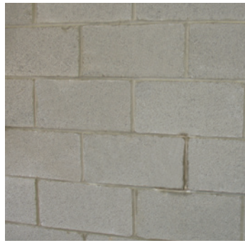
Project # 05-281 - After 72 Hours MasterPel 240-Treated Wall
