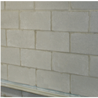
Project # 05-281 - Initial Testing MasterPel 240-Treated Wall
